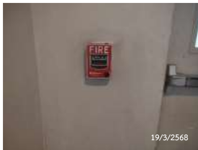
Fire Alarm Manual Station
